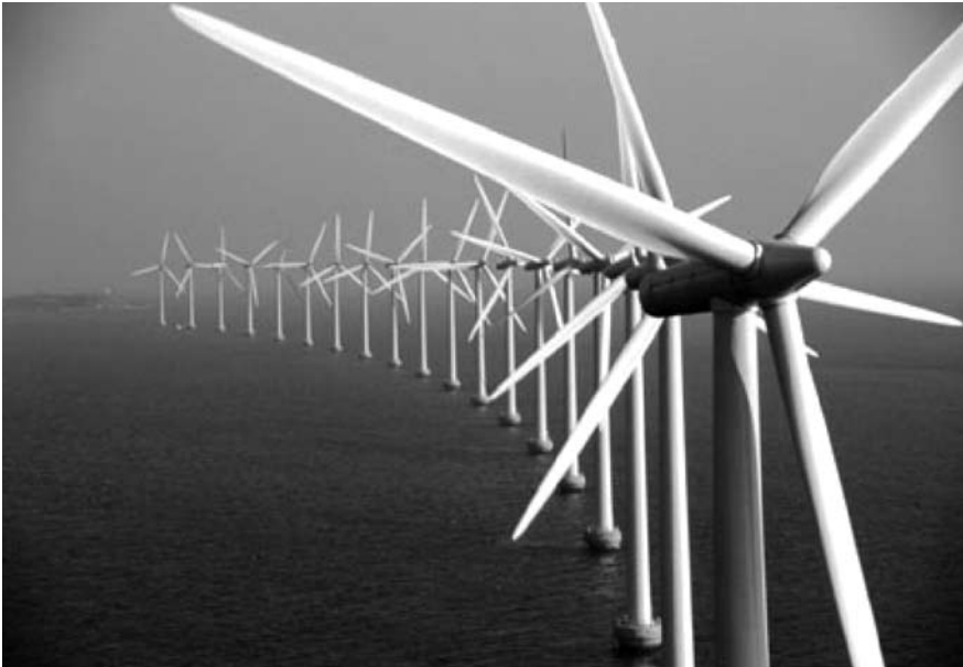
Figure 2.4: The Middelgrund offshore wind farm located just outside Copenhagen consists of 20 x 2 MW Bonus wind turbines (2000).
